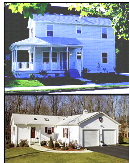
Examples of Desirable and Affordable Manufactured Housing with attached garages, appropriate roof pitch, front porches, and located on a foundation, crawl space or basement.
